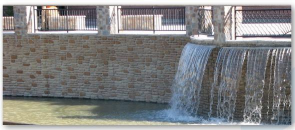
Formliners can be used with any concrete forming system to provide unique designs and economical solutions to forming architectural concrete surfaces.
