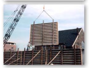
When you compare the Aluminum Beam Gang Forming System with other systems, you'll find that Symons offers a complete line of components and accessories to handle virtually any forming situation.
