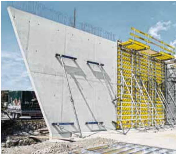
Outstanding concrete surface
