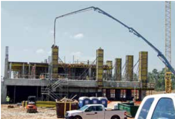
Precision Concrete Construction, Inc. utilized Doka's Frami column formwork to construct many of the stadium's exposed columns which required a smooth finish. Braves Stadium, Gwinnett County, Georgia
