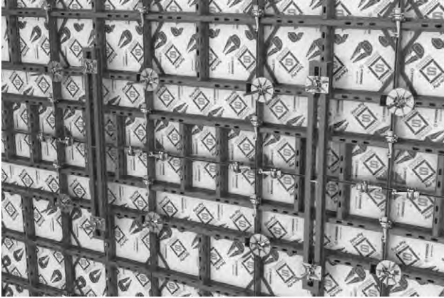
Stiffen Gangs with Sym-Waler (See Stacking Panels section for locations)
