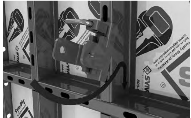
Aligner Bracket Installation
