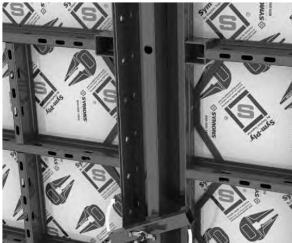
Turn Position Bar horizontal and hand-tighten the nut.
