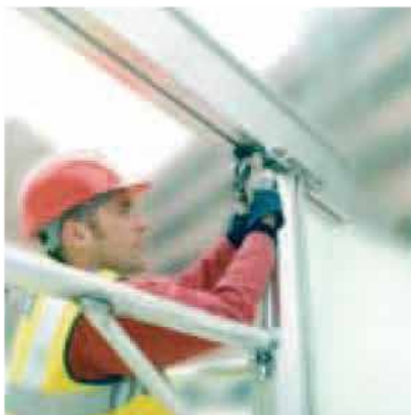
8. Fix primary beam to headplate by means of 2 R12 x 50 clamps.
