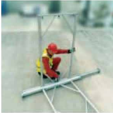
2. Connect ledger frame vertically to leg.
