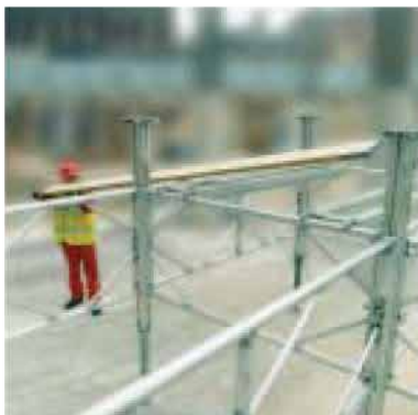
7. Place intermediate transoms and scaffold boards in position for fixing of alu beams.
