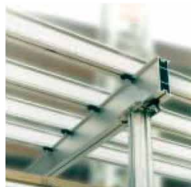
9. Position R12 x 100 and fix with a clamp at each intersection with a primary beam. Structure is now ready for fixing of plywood.
