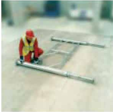
1. Connect ledger frame horizontally between 2 legs. Predetermined ledger frame position measured from headplate.
