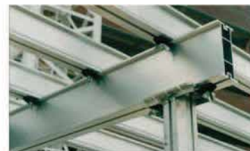
Headplate to beam fixing
