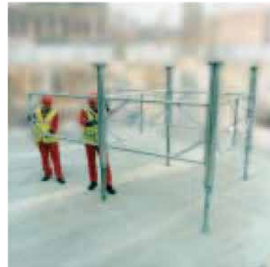
6. Now add additional frames and legs to form support structure.
