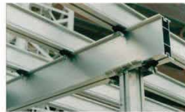
Headplate to beam fixing
