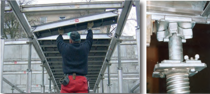
HV panel can be installed and removed from below.
