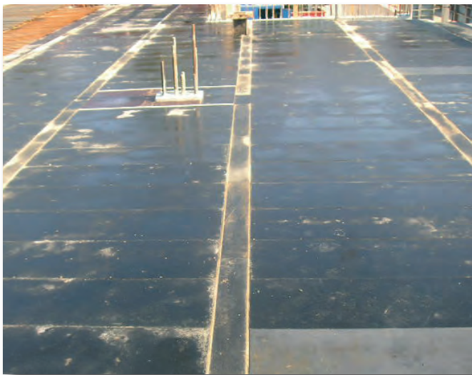
View of formwork surface with HV panels and HV filler strips
