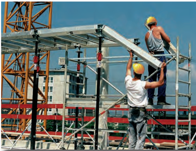
Hooking a main beam onto a drop-head.
