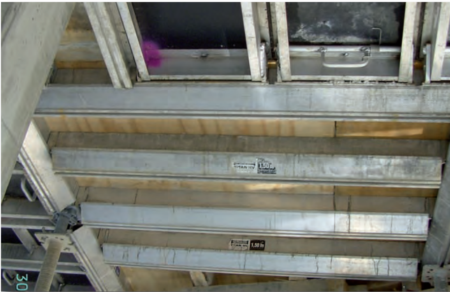
Make up panels with secondary or main beams and 3/4" plywood sheeting.
