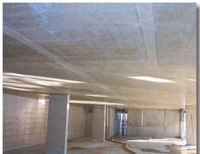
View of slab soffit with regular pattern of joints
