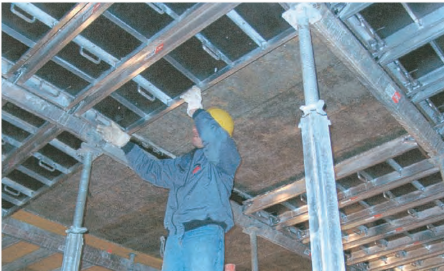
You can start stripping the formwork at any position.
