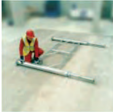
1. Connect ledger frame horizontally between 2 legs. Predetermined ledger frame position measured from headplate.
