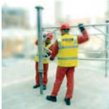
5. Connect both sides to form a 4 leg tower.
