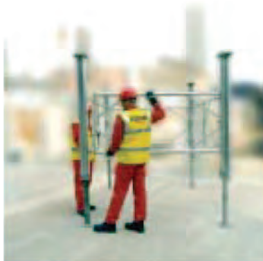
4. Repeat 1 to form 4th side of bay and then lift both sides of bay into position.
