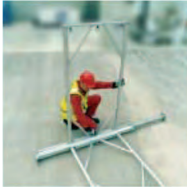
2. Connect ledger frame vertically to leg.
