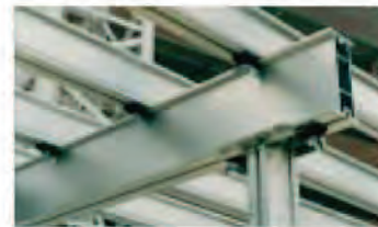
Headplate to beam fixing
