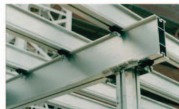
Headplate to beam fixing
